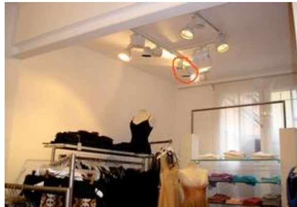
On the picture you can see a typical light installation which is very popular in shops. The camera is mounted into spotlight. You can adapt this easy to the rails system from the spotlights. In this version the camera is hidden by mirror glas. The 3011 allows you in addition to change the angle of view. So the spotlight housing faces to a different direction the camera is looking to.
