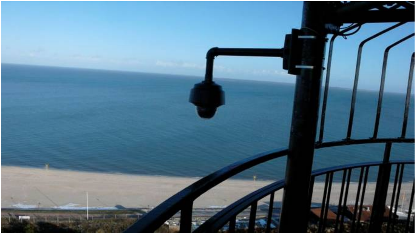
the new camera mounted to the antenna pole. Here you can see the new length of the wallmount.
